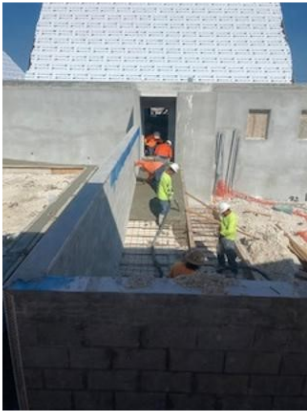
Pouring the ramp to the kitchen
